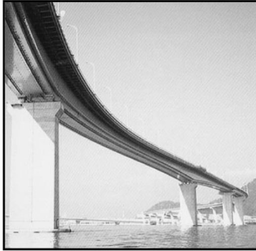
Figure 14. Kaita Ohashi Bridge with horizontal plate installed; (Japan Association of Steel Bridge Construction 1994)
